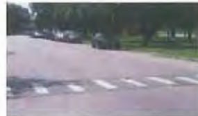
MARKED CROSSWALK Uses a visual cue to designate space for pedestrian crossings and alert drivers to priority crossing areas. PHOTO: Active Transportation Alliance
