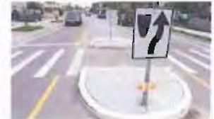
RAISED MEDIAN ISLAND Provides buffer and protection for pedestrians while crossing wide or busy streets. Adds space for green infrastructure. PHOTO: pedbikeimages.org/Dan Burden
