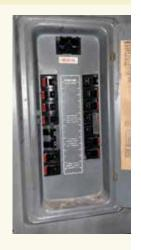
These circuit breakers may fail to trip in response to an overcurrent or a short circuit, possibly causing a house fire, property damage, and/or personal injury.
