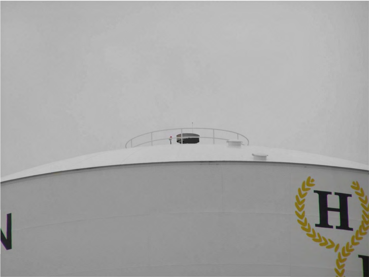
Beacon Pointe Water Tower
