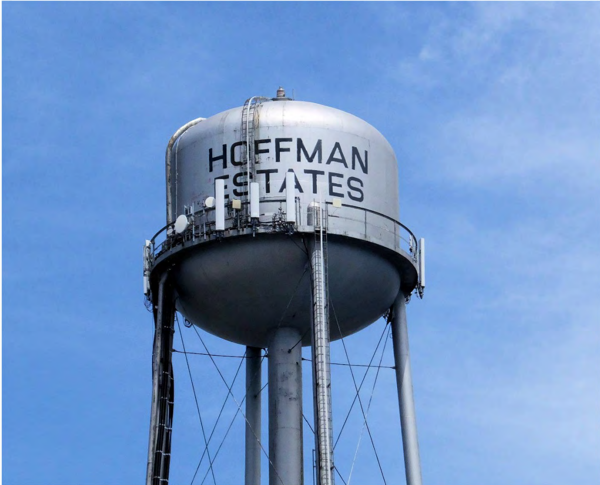
Aster Water Tower
