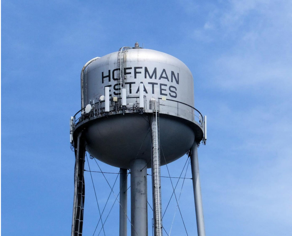
Aster Water Tower
