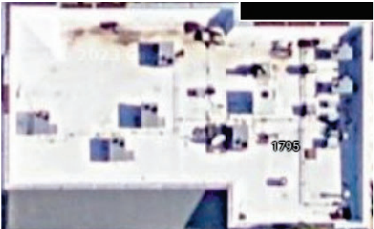
AERIAL PHOTO OF EXISTING ROOF
