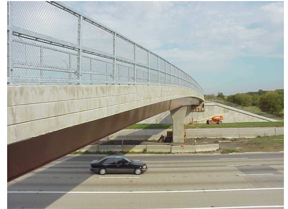
Figure 44. I-290 Overpass Bicycle Bridge
