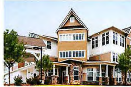
STONECREST OF CLAYTON VIEW Saint Louis, MO
