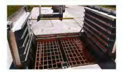
Lift station type: Sanitary Sewer Triplex Submersible Lift Station Lift station capacity: 1,307 GPM @ 26' TDH 2 x 27 HP Pumps
