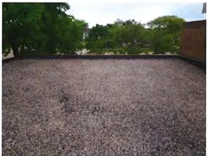
south wall has coping
