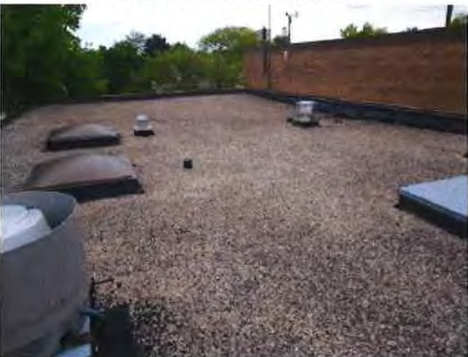
lower roof for cores
