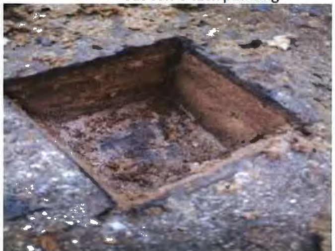
cut 1: deck runs north-south bottom-up: 5/8" drywall, 2-ply, 0.5" fesco, 1.5" iso, two layers of hardboard ~1-5/16", four plies B.U.R.
