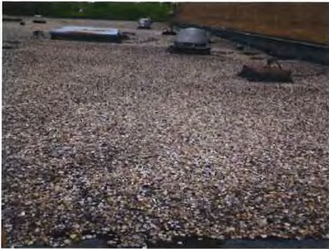
2 drains at wall
