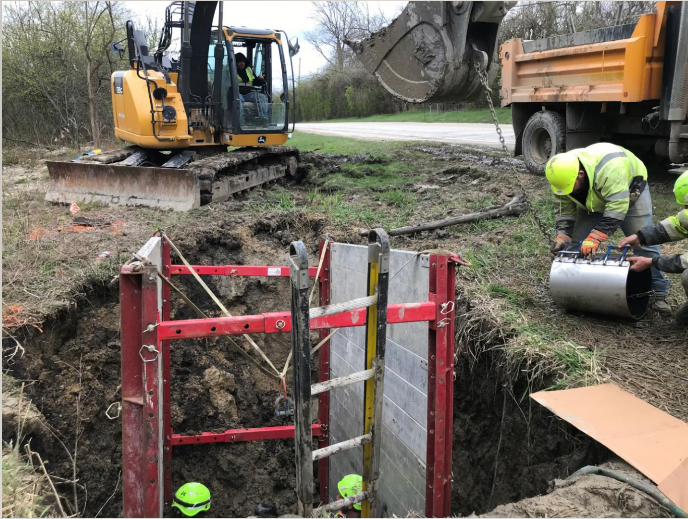
Water Construction staff place a repair sleeve on a leaking water main.
