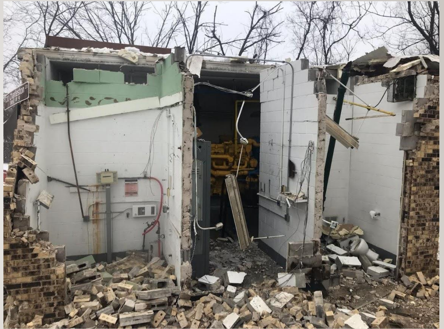
Demolition of a well-house for a decommissioned well.
