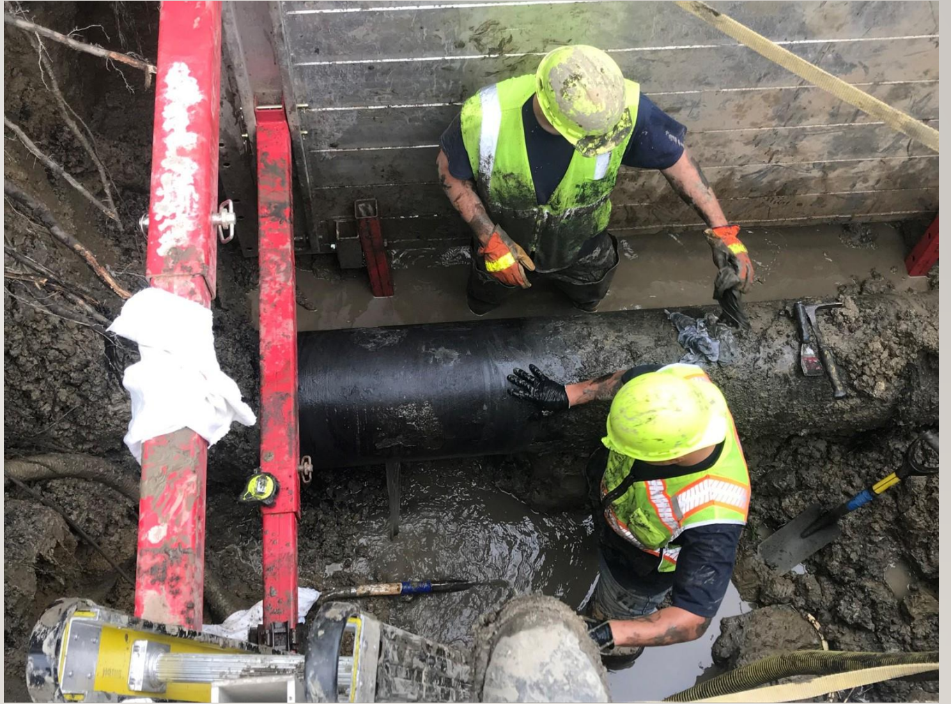
Water Construction staff excavate to repair a leaking water main.
