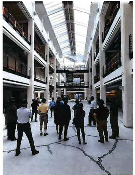
Figure 1: On September 2nd, members of the Village Board and Staff toured the progress of Bell Works, led by Ralph Zucker of Somerset Development.
