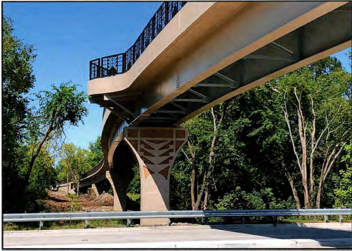
Looking north – Bike Bridge over Central Road
