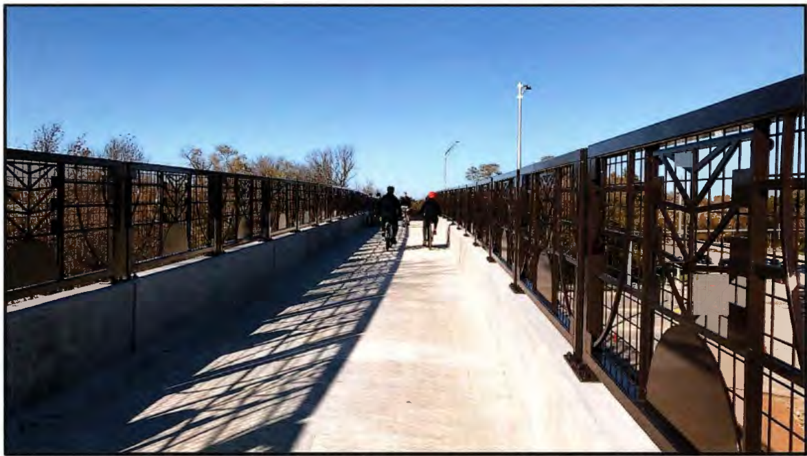
Looking north on new bridge over Central Road
