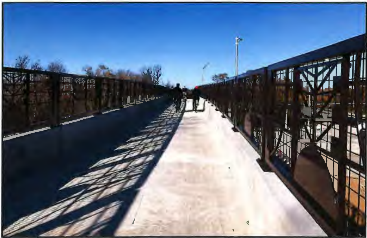
Looking north on new bridge over Central Road
