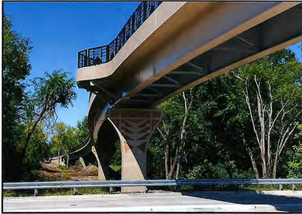
Looking north – Bike Bridge over Central Road
