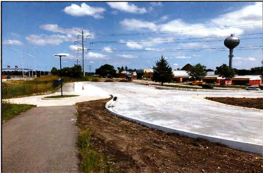
Pace Kiss-n-Ride Construction – Looking southeast towards Pembroke Avenue
