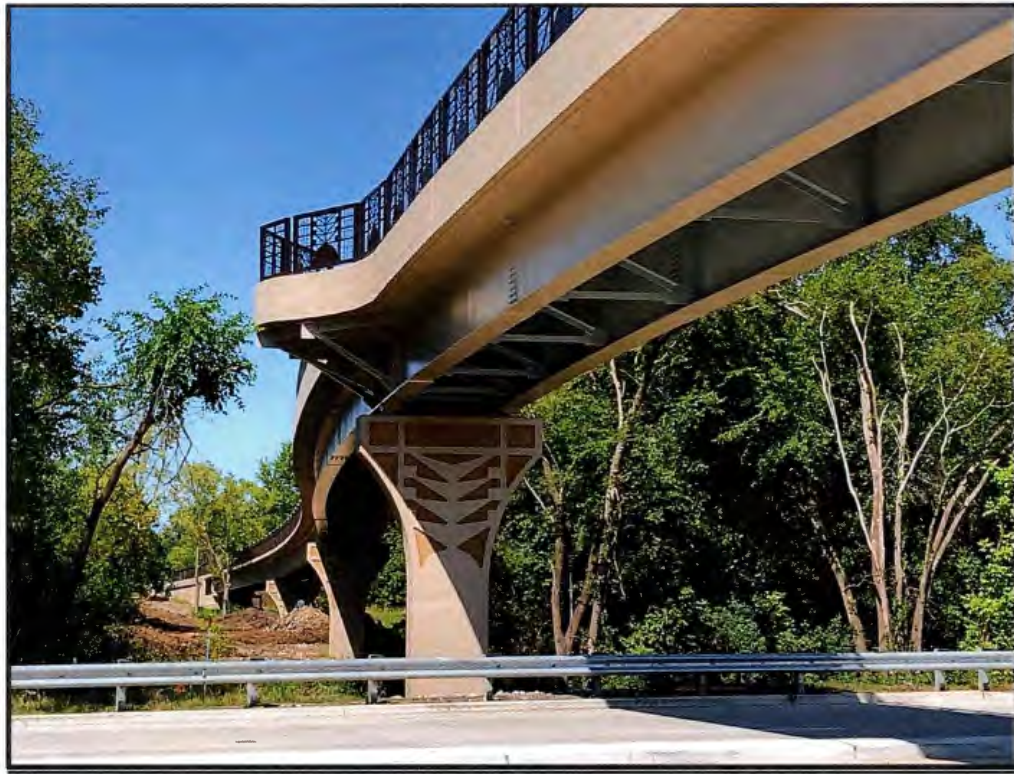
Looking north – Bike Bridge over Central Road
