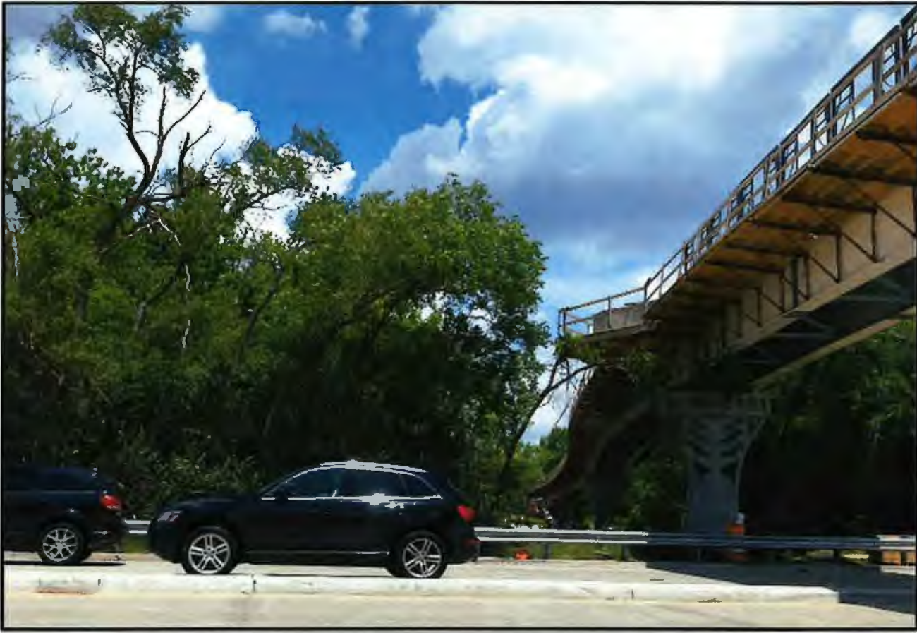
Looking north on Central Road – Bike Bridge over Central Road
