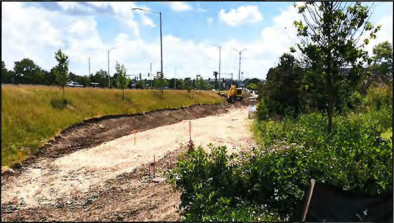
Looking south towards Hillcrest, west side of Roselle – south of I-90
