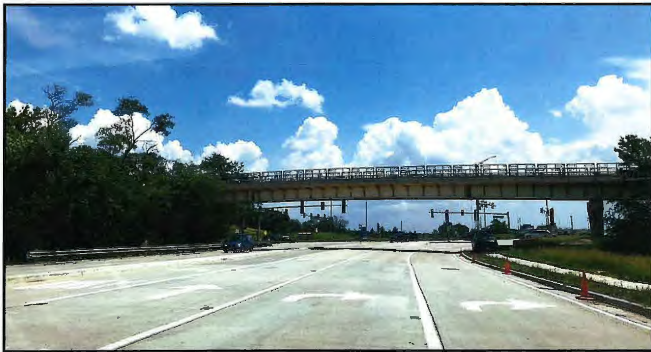
Looking east on Central Road – Bike Bridge over Central Road
