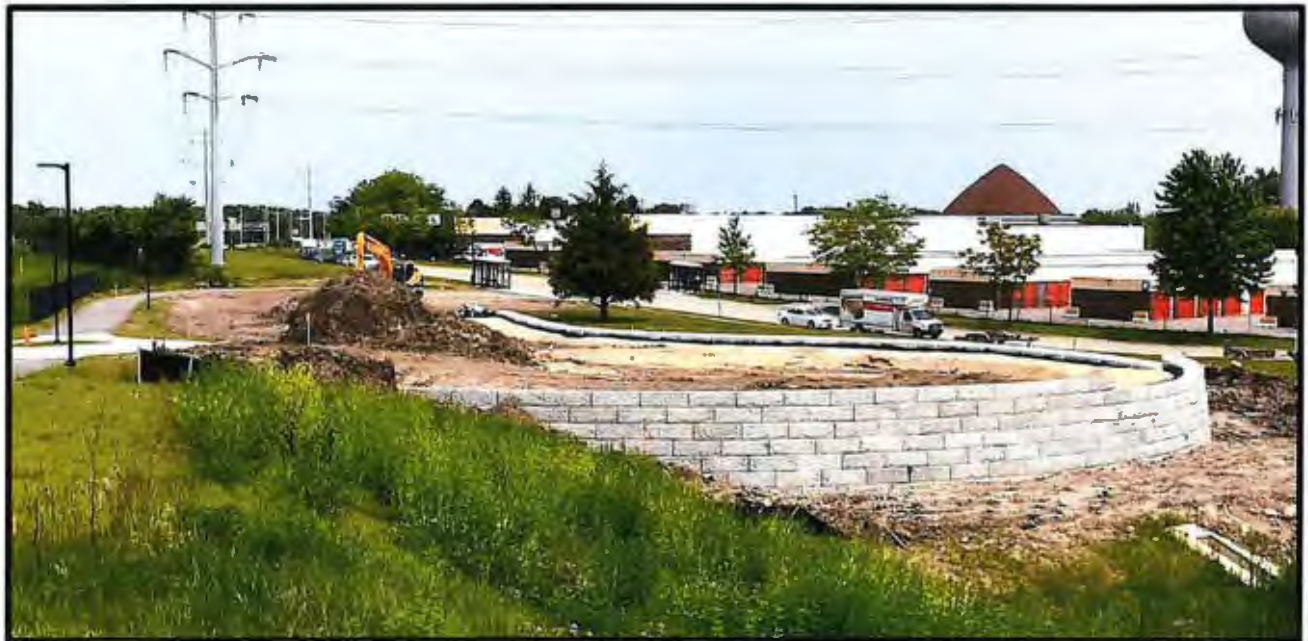
Pace Kiss-n-Ride Construction – Looking southeast towards Pembroke Avenue
