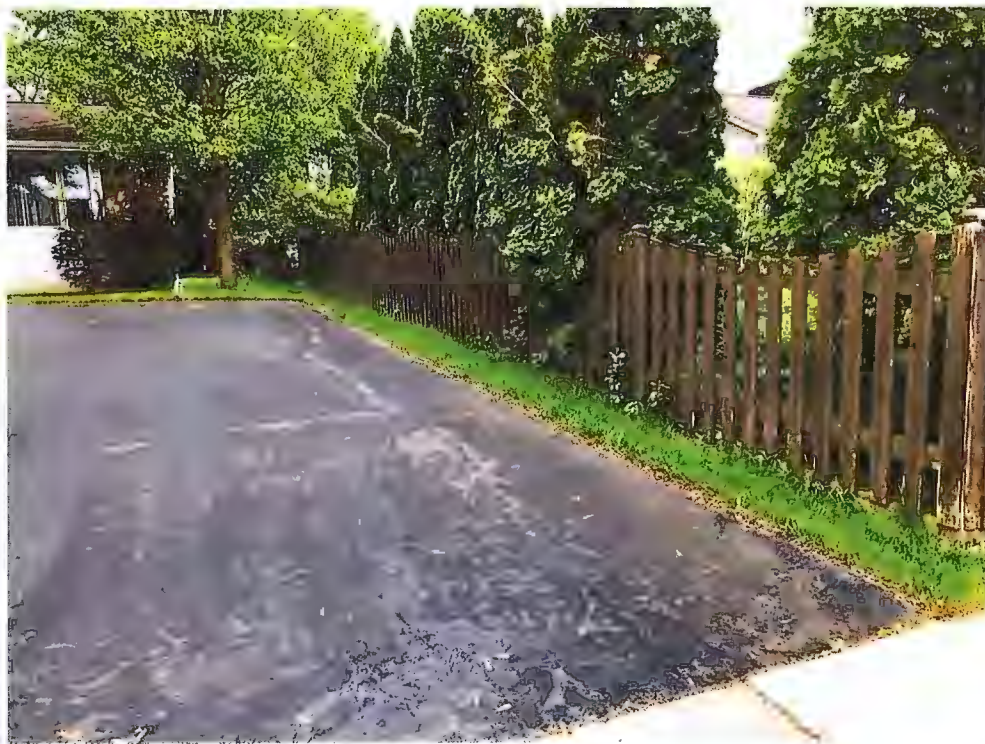
Back Rear Corner (3928 Driveway)
