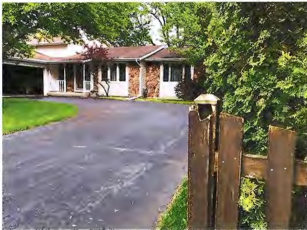
Rear Corner (3928 Driveway)
