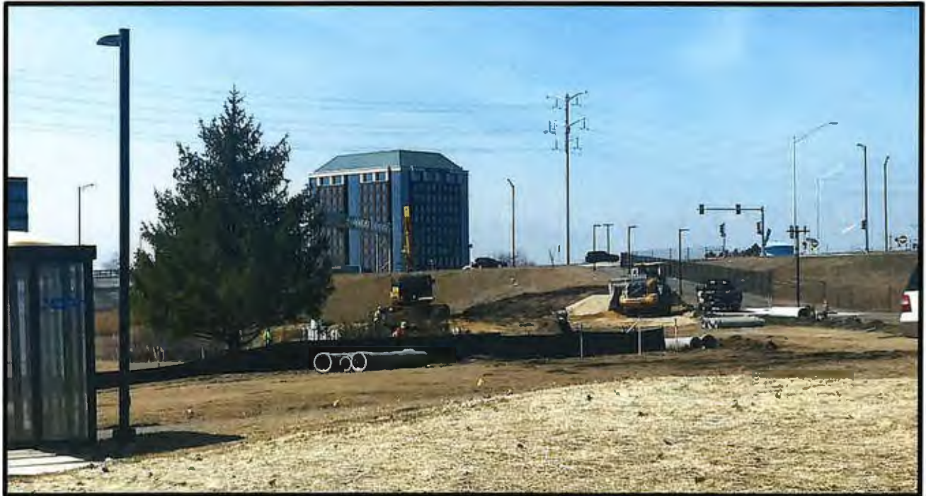
Pace Kiss-n-Ride Construction – looking northwest from Pembroke Avenue
