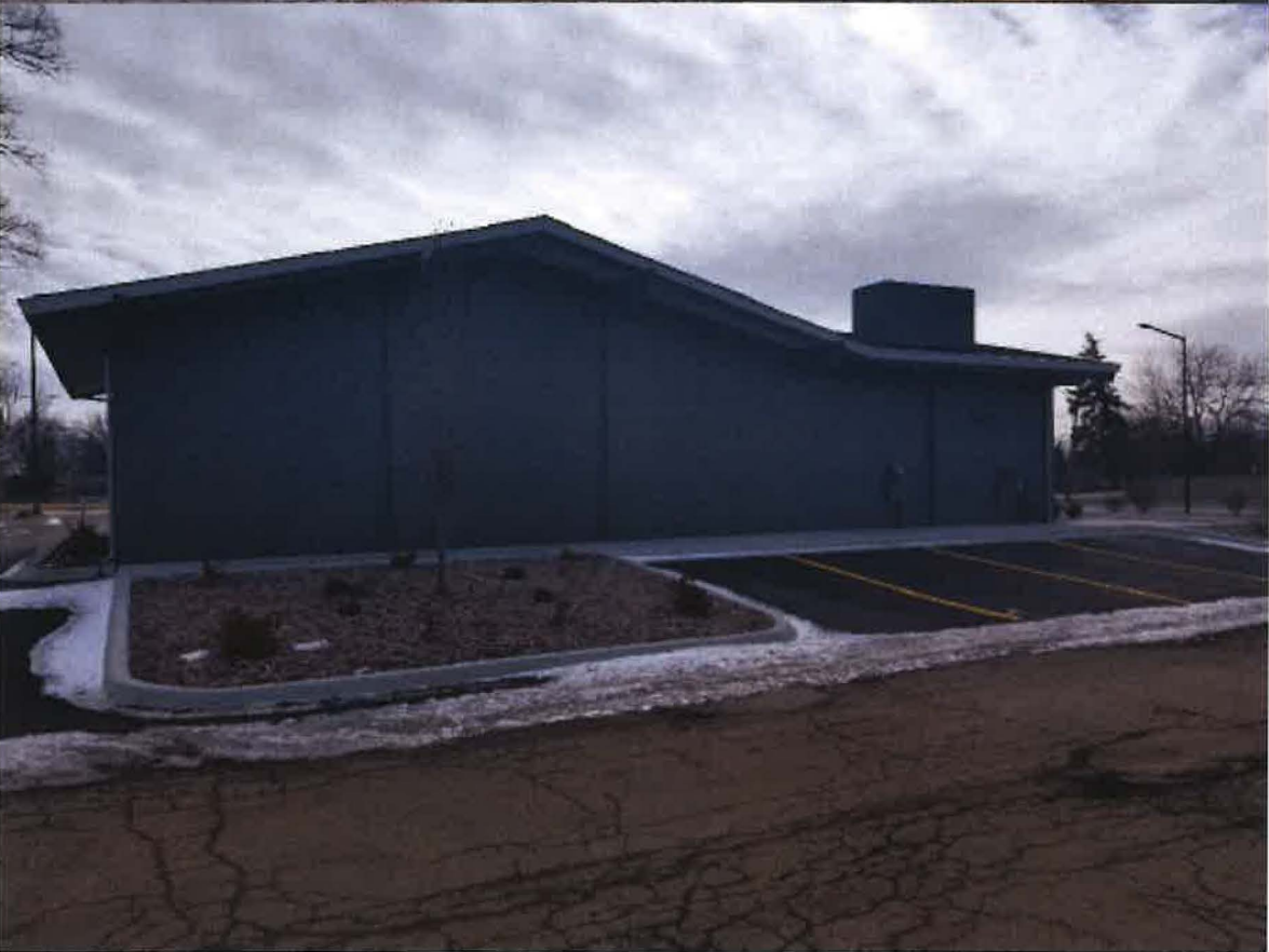
North (rear) Elevation - AFTER
