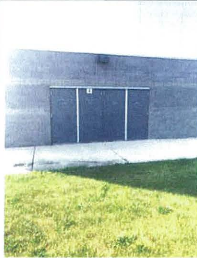
Emergency Exit Doors
