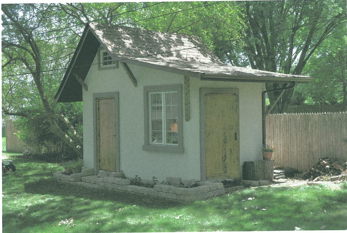
Front & side view of the shed.
