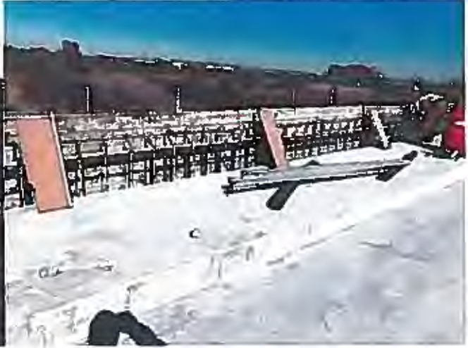
Framing and Rebar Installation
