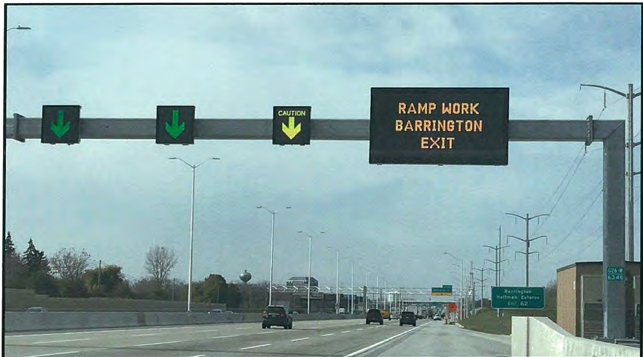
SMART Road Technology Sign Gantry, Information Panels, and Lane Control Signals
