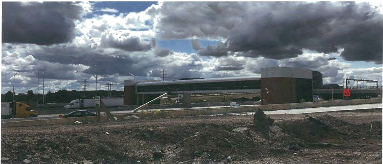
View of pedestrian overpass and buildings from Park-n-Ride area
