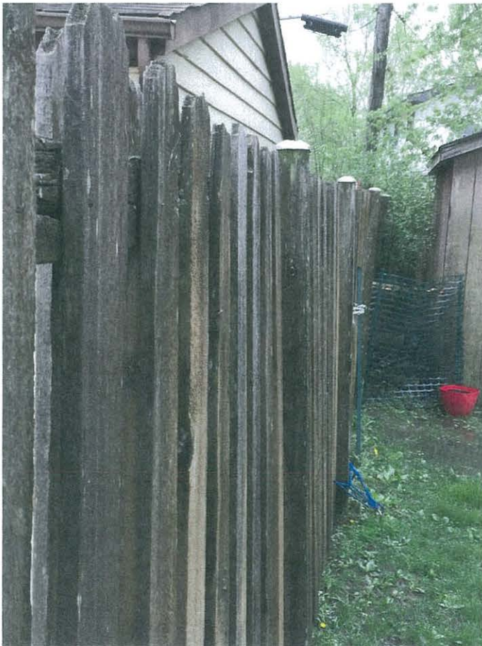
Eastern side of Fence.
