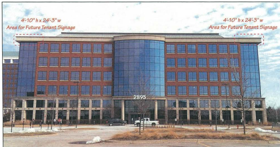
2895 W. Higgins Road - West Elevation
