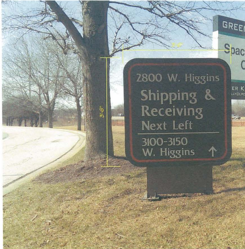
Existing (1) 3'-6" x 3'-6" Non-Illuminated Post & Panel Directional Sign
