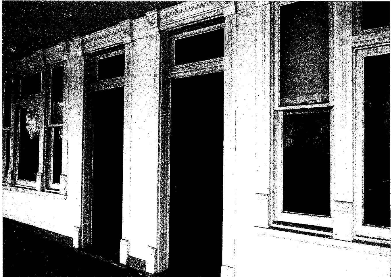
ENTRANCES FROM PORCH TO THE FRONT PARLOR
