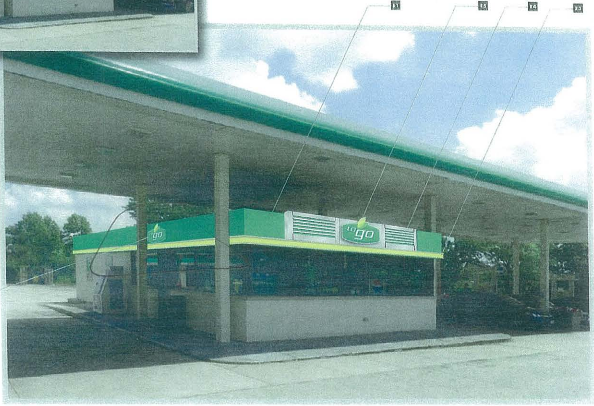
Front and two side are the same with green ACM and dimensional awning
