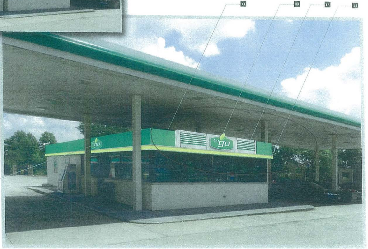
Front and two side are the same with green ACM and dimensional awning
