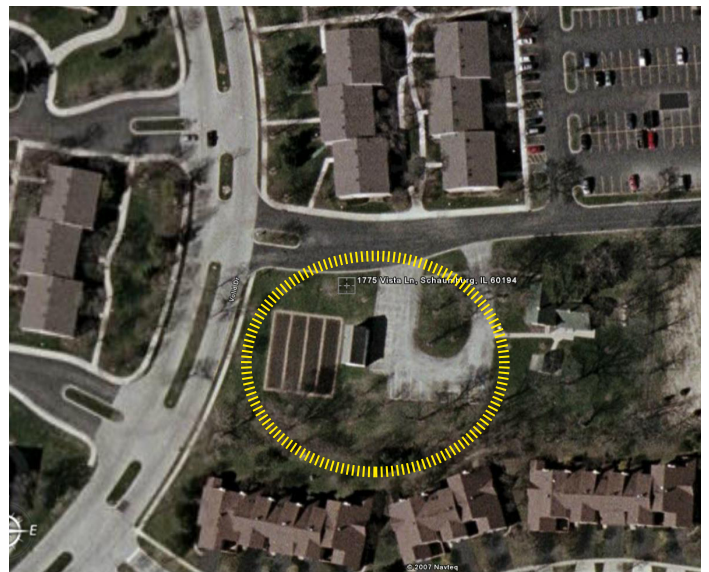
Figure 6.14: Aerial view of the Sunderlage Farm House
